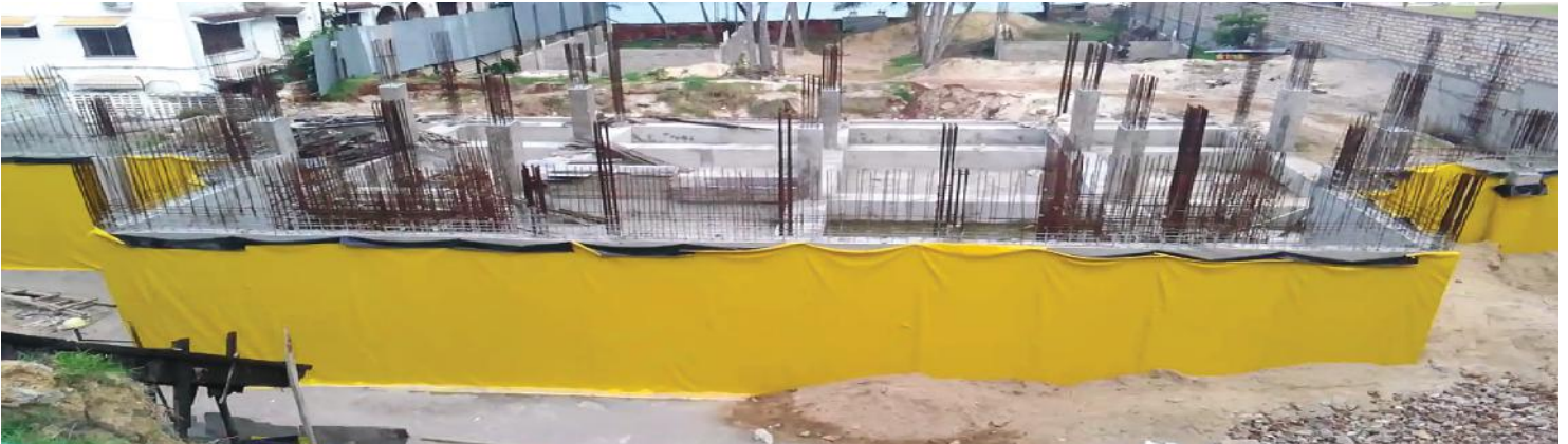
Nyali, Mombasa Project
